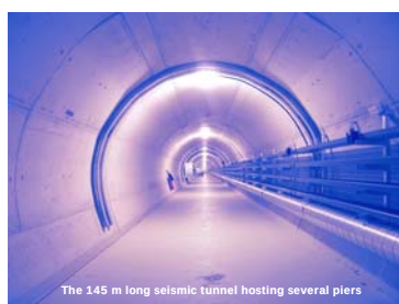
The 145 m long seismic tunnel hosting several piers
